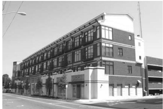
Figure 10.12 Apartments screening parking deck. Park Avenue, Charlotte, NC, 2002. David Furman, Architect. The parking deck is shared with an adjacent office building and street level stores. This is a standard, but highly effective urban typology. The only drawback is that the apartments are single aspect, that is, they face only one way and are accessed off an internal corridor. The consequent lack of natural cross-ventilation means that most climate control has to be mechanical even under benign external conditions.
