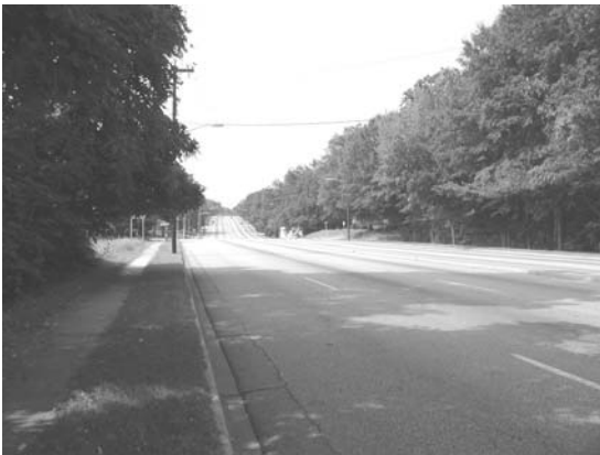
Figure 10.11 Site of Church Street Neighborhood Center, as existing (Compare with Plate 42).
